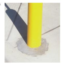
installation. Once the concrete is cored and the bollard is in place, the hole must be backfilled with concrete to secure the bollard in place. For added strength, these bollards are often filled with concrete, as well. Though the bollard pipe itself is relatively inexpensive, this installation method is costly and time consuming.
