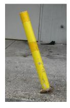
The downside to this installation method, when used with a rigid bollard, is that the anchors are generally not strong enough to withstand anything more than a minor collision. The plate anchors often are pulled up and possibly the plate bends, leaving a post which leans and is no longer able to properly serve its purpose. Plate mounted bollards often require constant maintenance and replacement.
