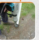
1 Stand post in position for installation 2 Insert driver tool into the spike sleeve 3 Hammer post into ground until top of spike is level with surface
